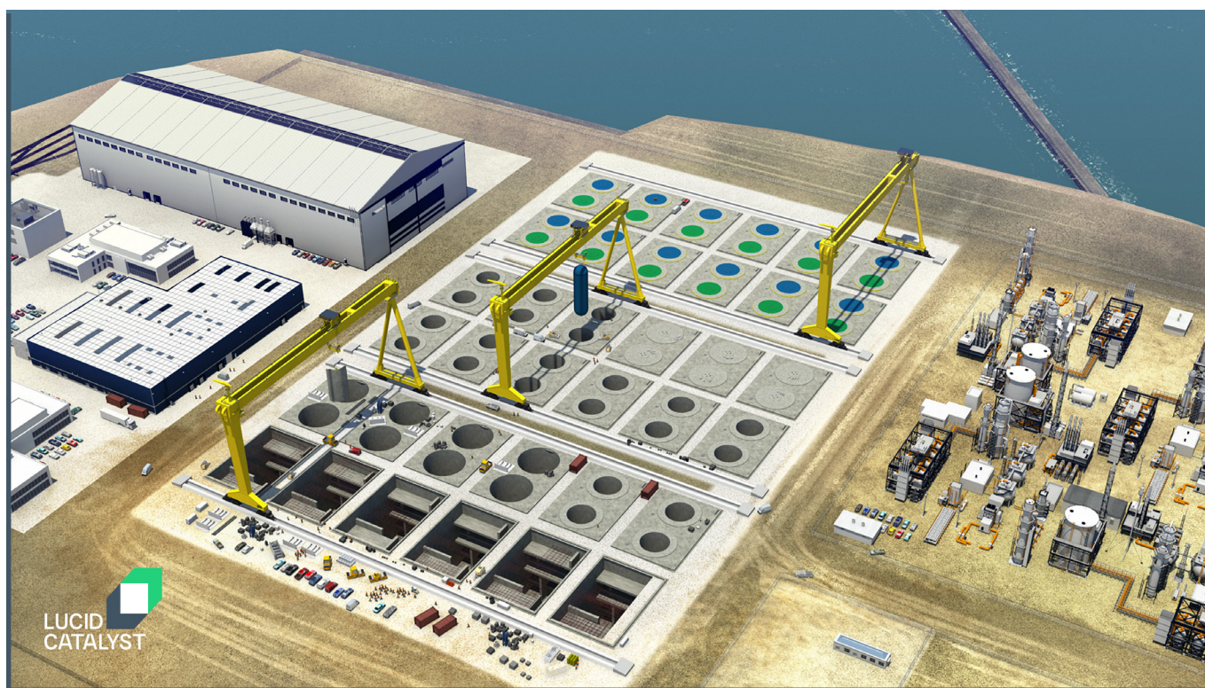
Figure 13. Another view of a hydrogen Gigafactory under construction
